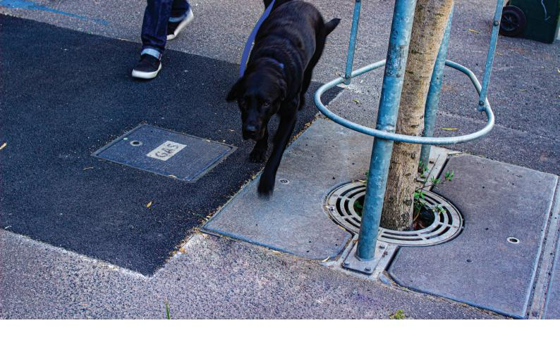
Regular maintenance needs meant lids designed for infill pavers were not a practical solution due to excessive weight. This problem was exacerbated by the close proximity to the ground of the tree guard making it impossible to place lifting gear above the lids.
